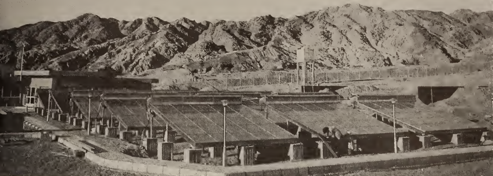
Solar energy plant near Al Aqabah
